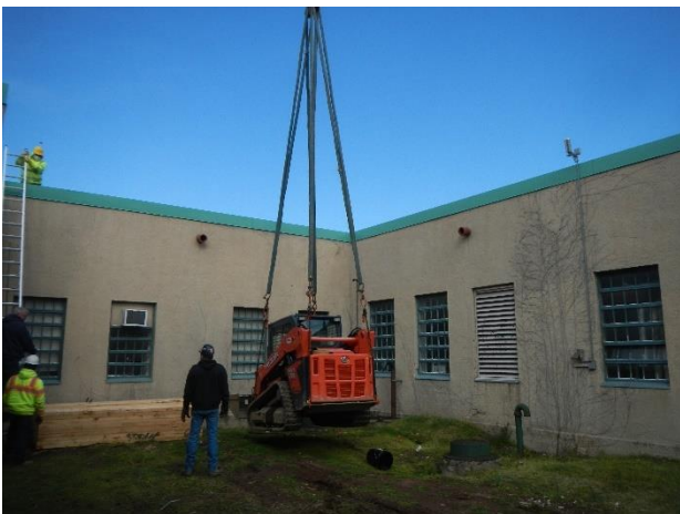
A crane was required to access the problem area
