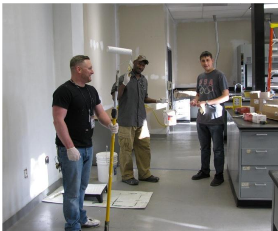
Vance, Keith, and Mariusz getting ready to prime the walls.
